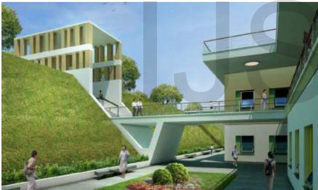
Fig: 7 Earth Sheltered building at BITS PILANI Campus
